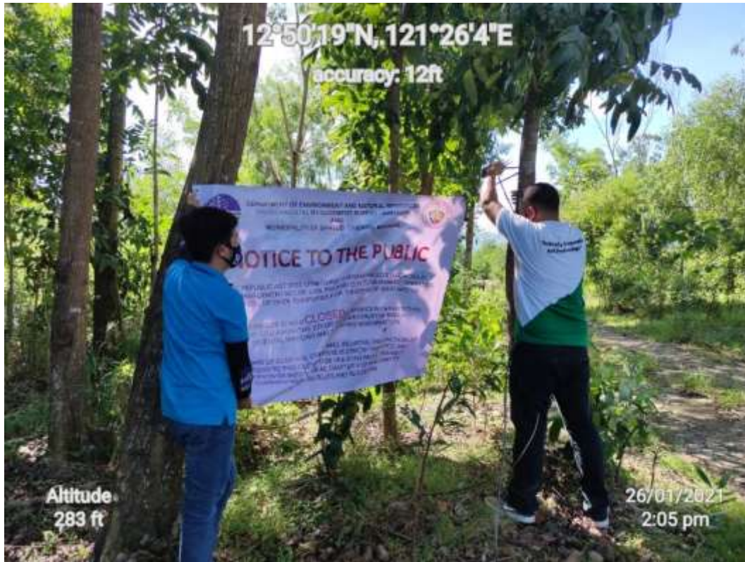
Installed Signage/Tarpaulin for the Permanent Closure of LGU Bansud Dumpsite
